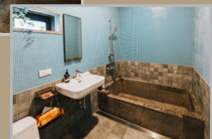
▲ 重新打造的傳統磨石子浴缸，出自執業數十年的南部老師傅之手。 The traditional terrazzo bathtub was custom-built by a southern Taiwanese artisan with decades of experience.
