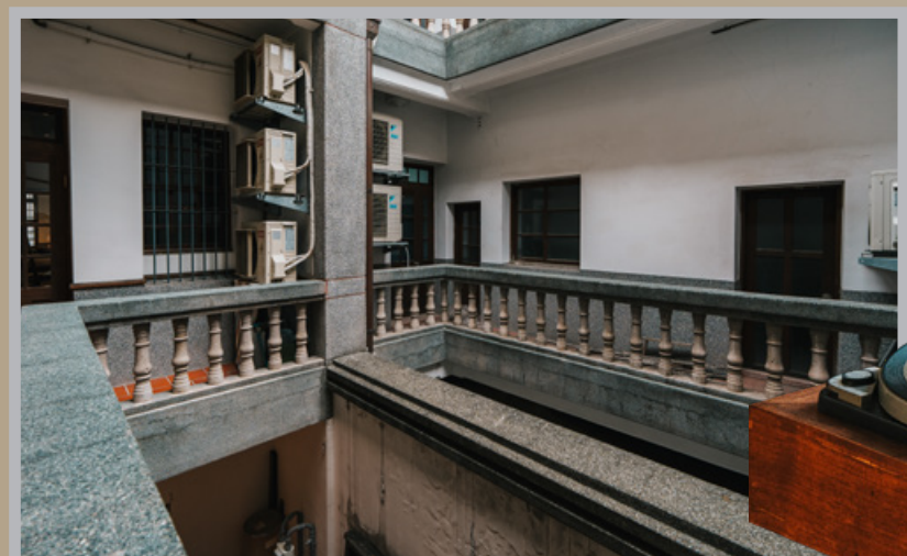
▲ 以「洗石子」工法製成的天井牆面 The courtyard walls are finished using traditional terrazzo techniques.
